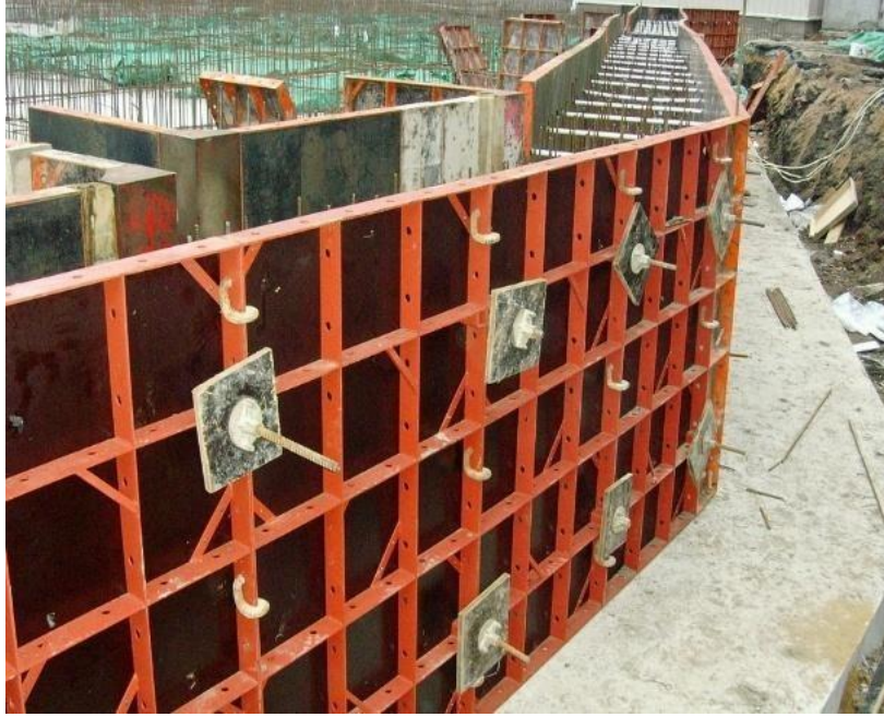
Figure 3.7 – Scheme of small-panel formwork
